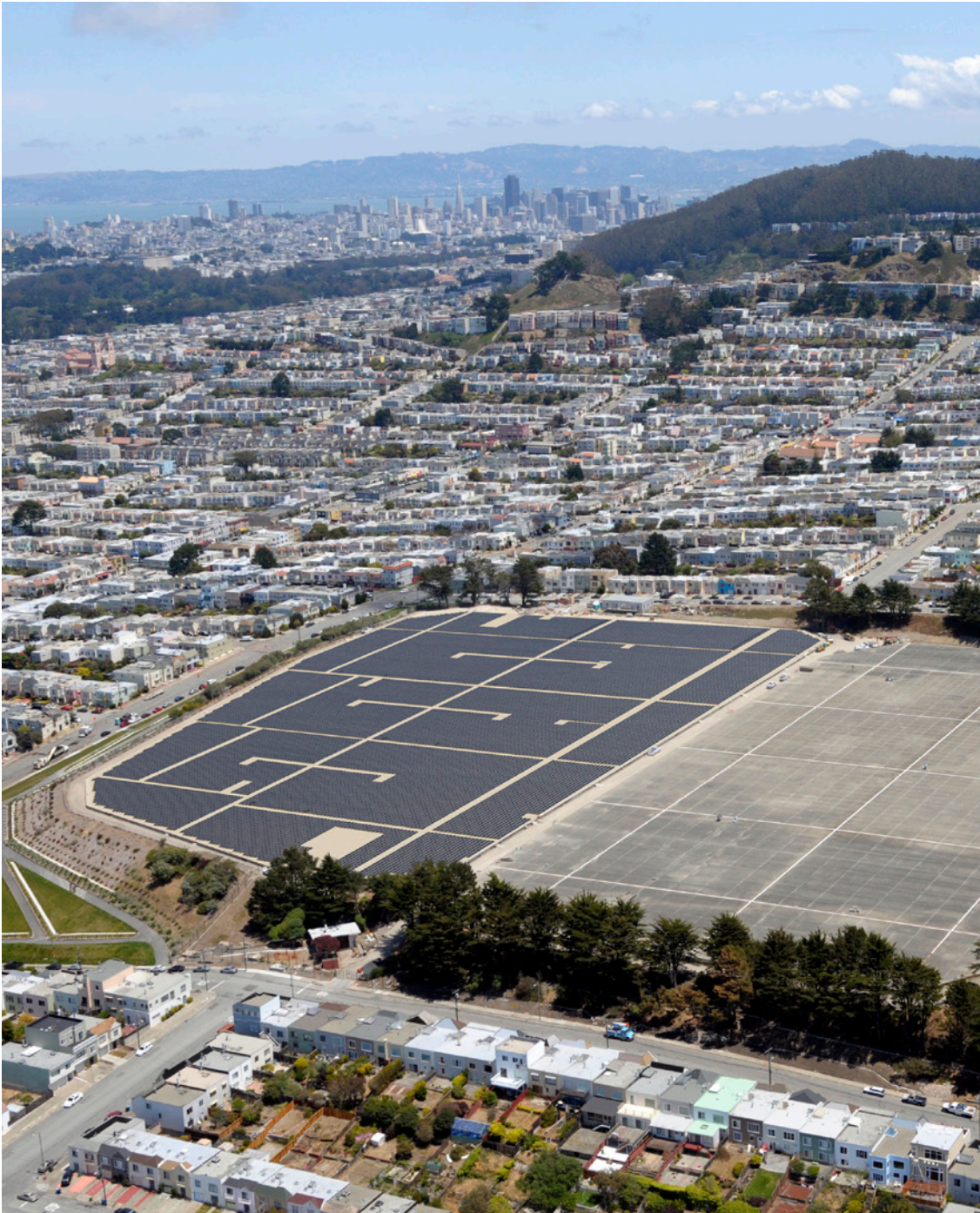
Aerial view of Sunset Reservoir with digital rendering of solar array
