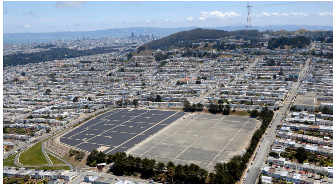
Aerial view of Sunset Reservoir with digital rendering of solar array
